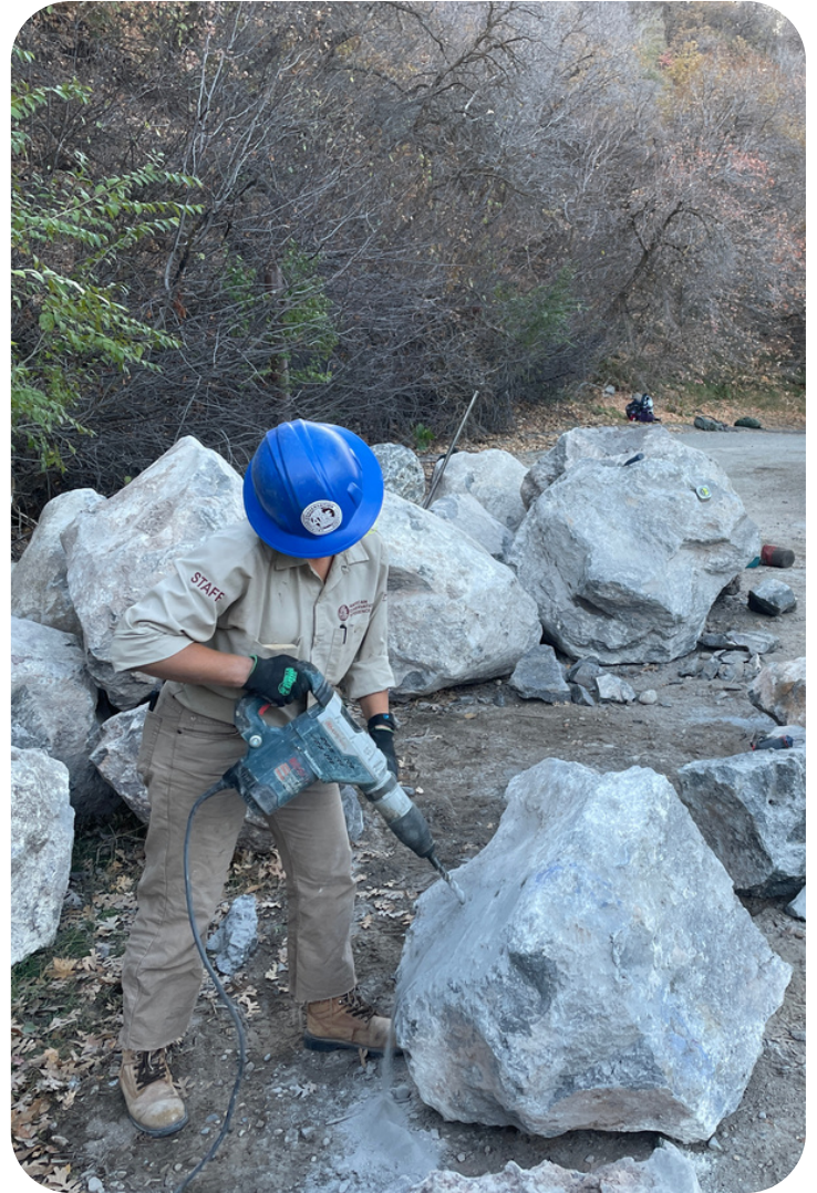
Top Left: Assistant Team Leader Brandi Marlett using shaping hammers to shape a step rock to better fit its hole.
