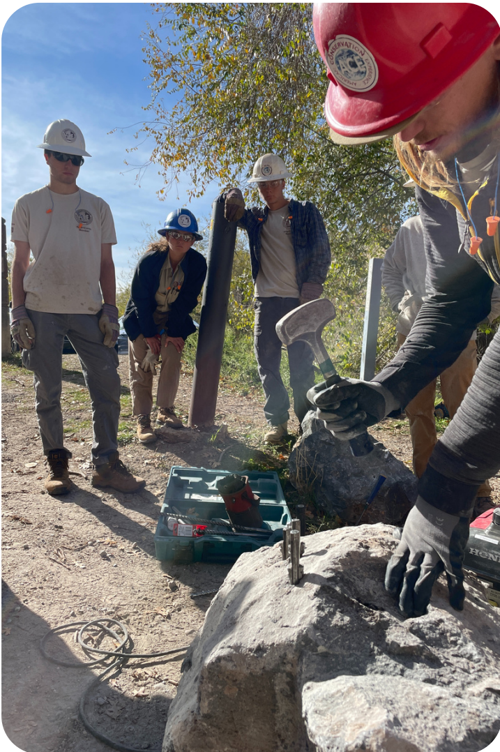
Top Right: Crew Leader Casey Bainbridge using a rock drill to prepare a boulder for shaping into steps and gargoyles.
